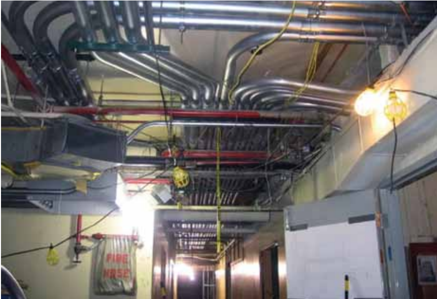
Conduit Bends, Scott Demel (Local 3 Electrician)
